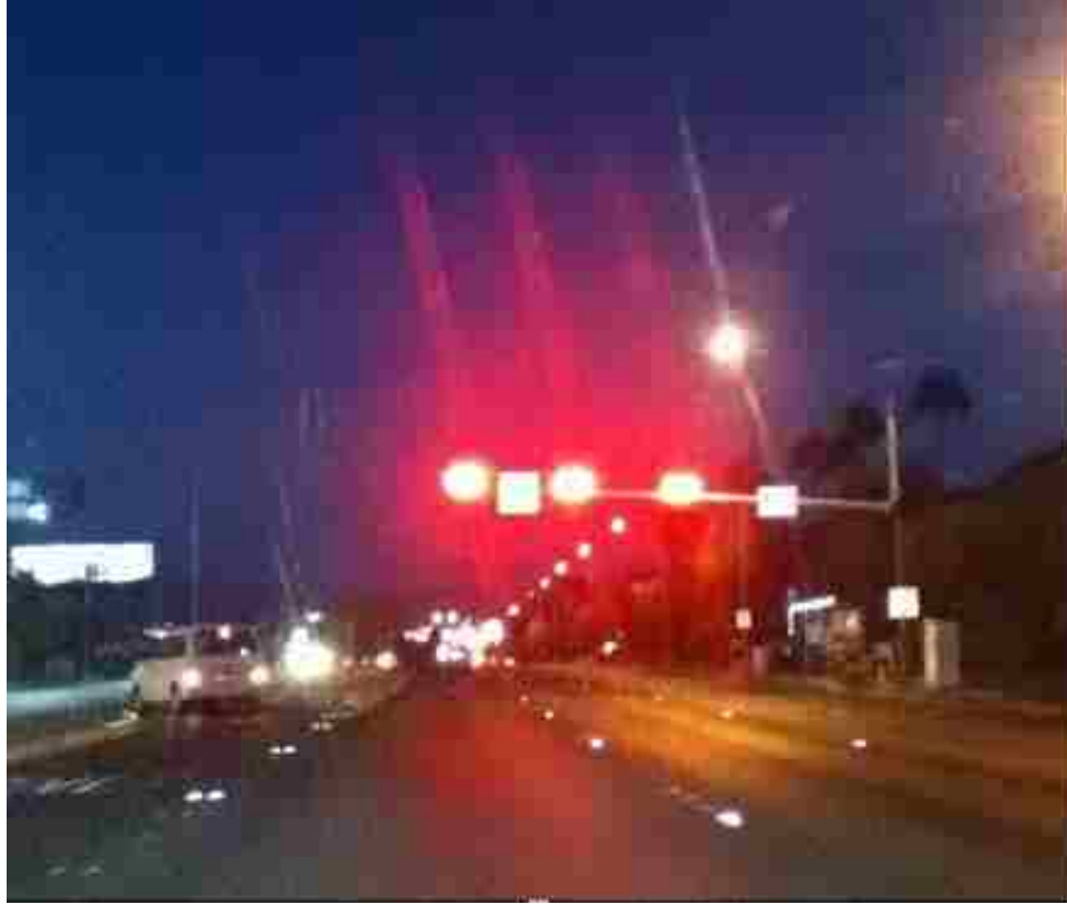
Figure 3-13. View of Activated PHB System at Night
